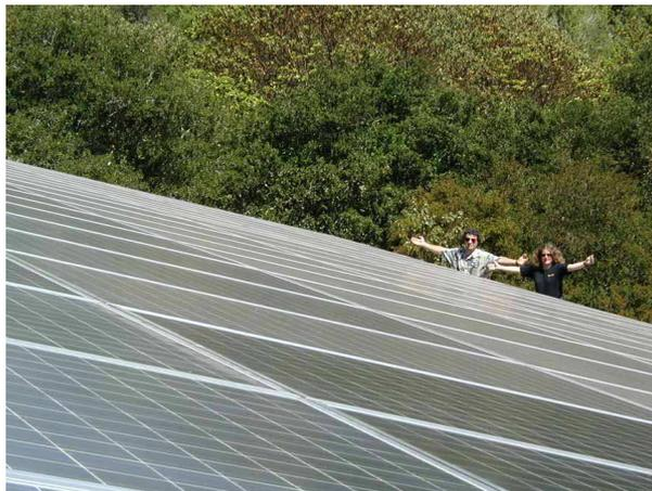
**Figure 22:** An array of solar panels near Santa-Cruz ([www.solarwarrior.com](http://www.solarwarrior.com)). The panels cover  $220\text{m}^2$  and supply an average power of  $5\text{kW}$ .
